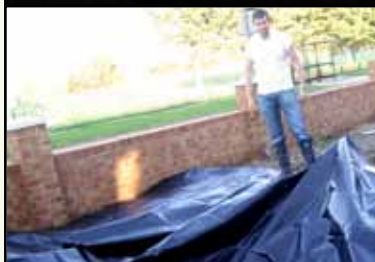
Opening liner out
