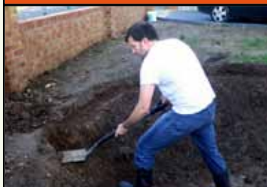
Digging the pond
