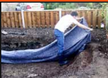
Lining with underlay
