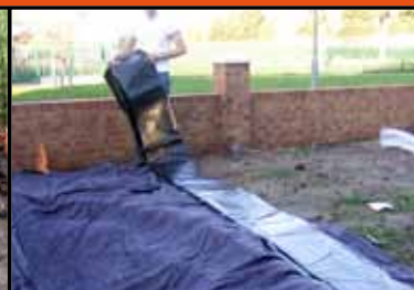
Rolling out the flexiliner
